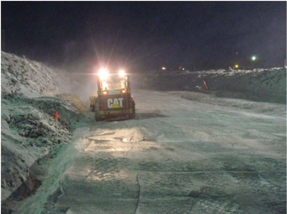
Photo 12: Skid steer with brush cleaning edge of transition material on the downstream edge of the key trench.
