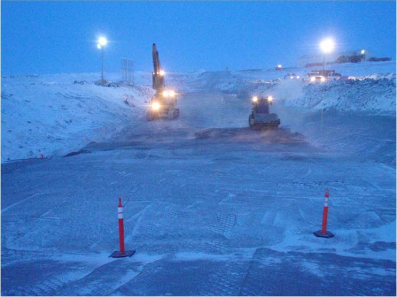
Photo 6: ~ENE view of FCM placement around station 1+10. The delineators in the forefront of the photo mark the area where FCM placement started on dayshift.
