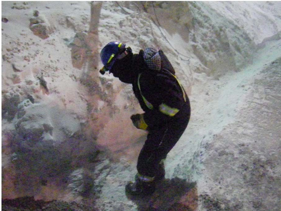
Photo 11: Labourer cleaning snow from the trough along the downstream side of the key trench.
