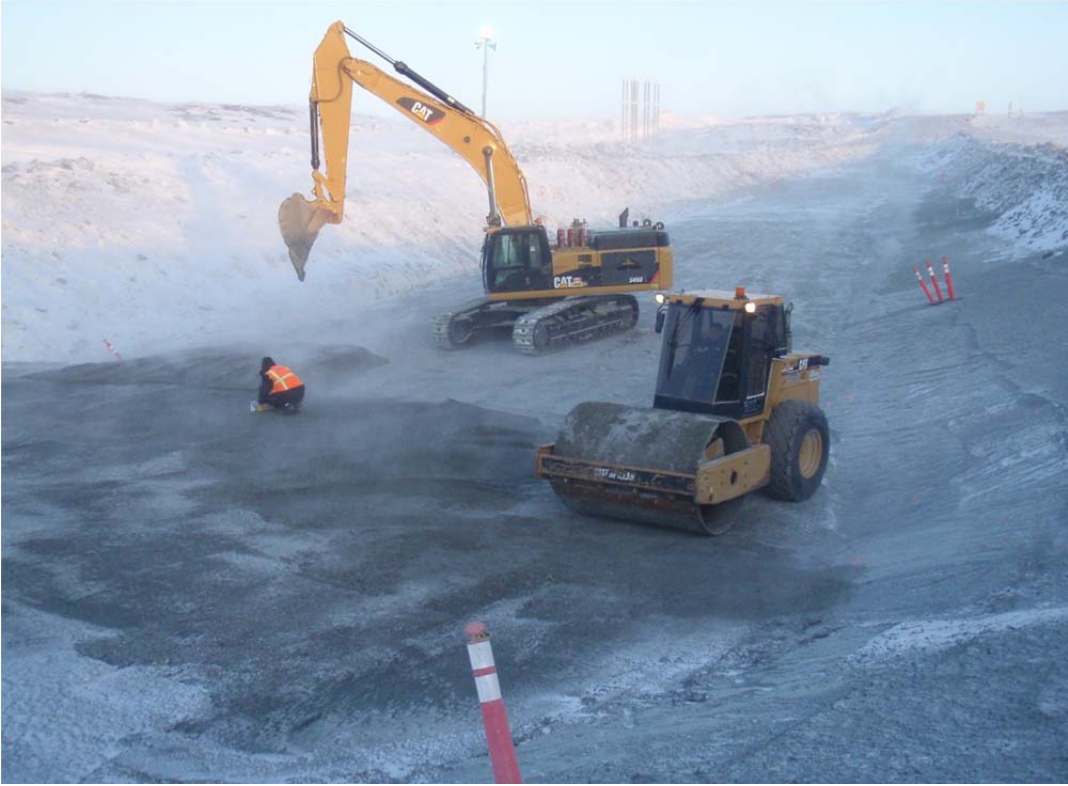
Photo 4: ~NNE view of FCM placement progress around station 0+90.
